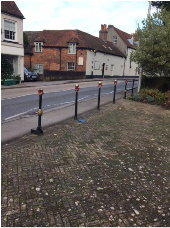
(blue book indicating loose bollard)
