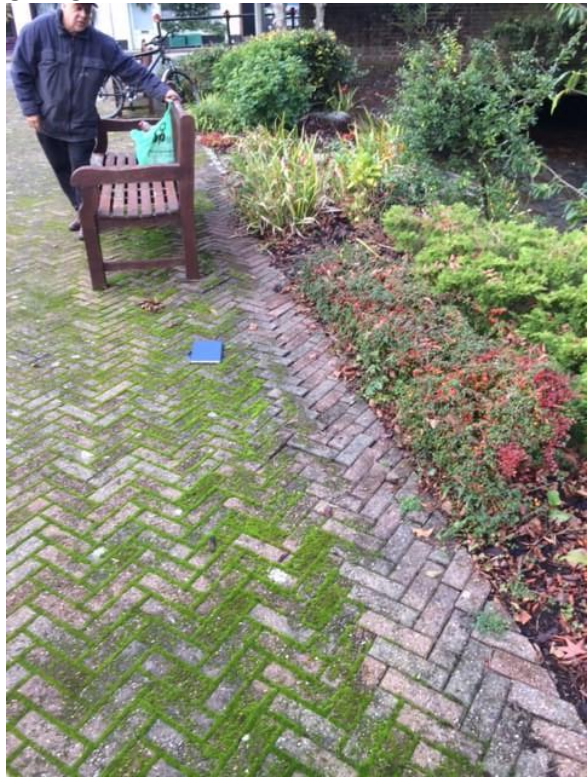
Block paving faults (note blue book as indicator)
